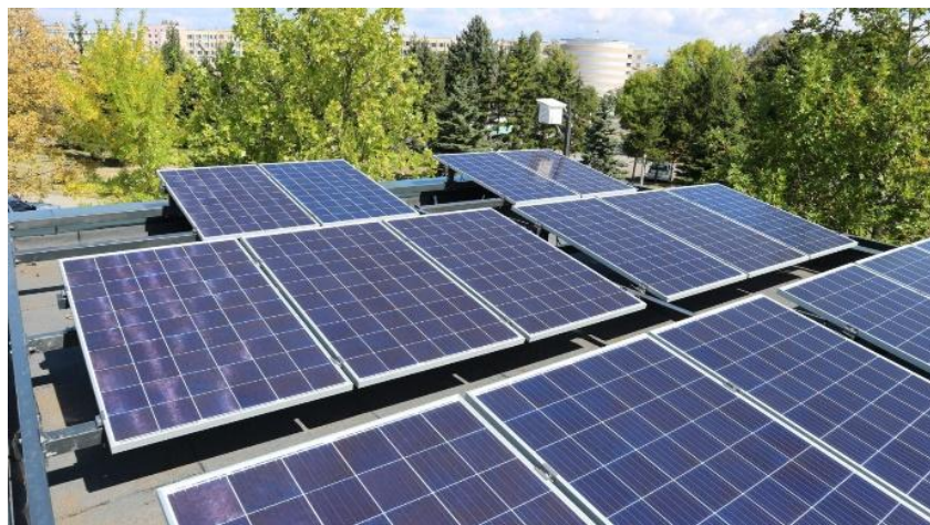
Figure 3: PV system on the roof of the innovative demonstrational Pavilion in Sofia with installed capacity 5.04 kWp.
