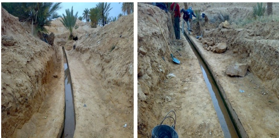
Figure 5: Rehabilitation of the seguias of the Béni Ounif oasis (2008)
