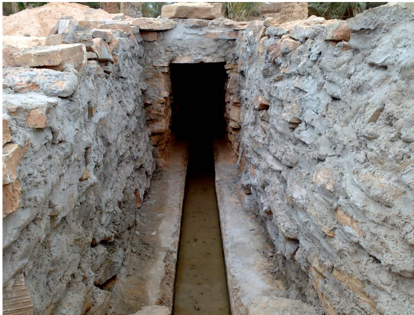
Figure 3: The outlet at the exit of the Béni Ounif foggara (2008)
