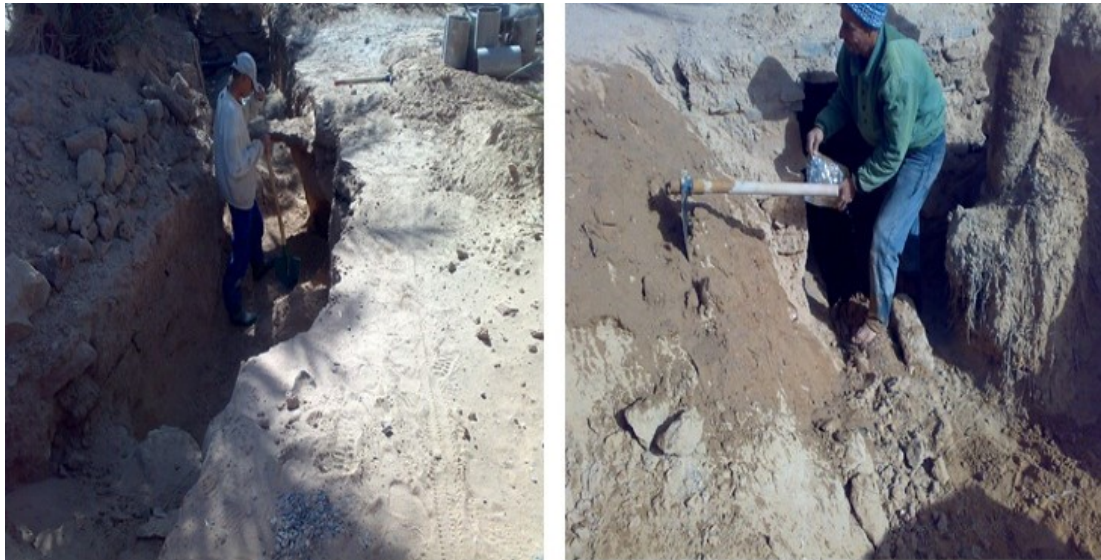
Figure 4: The rehabilitation works of the foggaras of Béni Ounif (2008)
